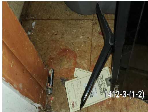
1412-3 9"x9" Floor Tile/Tan (3% Chrysotile) Mastic/Black (2% Chrysotile) Interior Hall Closet (15 sq. ft.)
