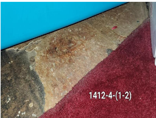
1412-4 12"x12" Floor Tile/Tan (2% Chrysotile) Mastic/Black (2% Chrysotile) Interior Bedroom B (15 sq. ft.)
