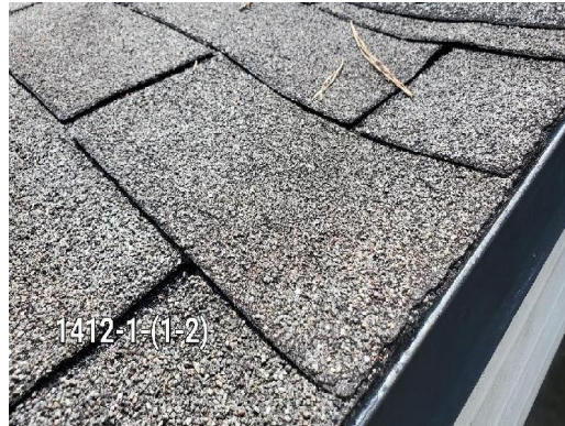
1412-1 Asphalt Shingle/Gray, Tar/Black Typical Exterior Roof
