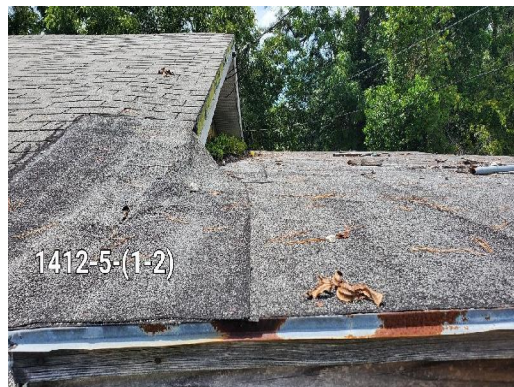
1412-5 Rolled Roofing/Gray Typical Exterior Roof
